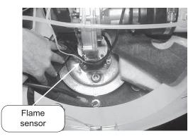
Step 8. Install new flame sensor with new gasket provided using screws from step 6. Arrange flame sensor with hook towards burner.
